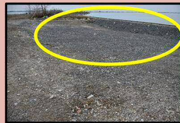
Existing soil from the pier's West edge was used to fill in pit test holes, weakening the edges further.
